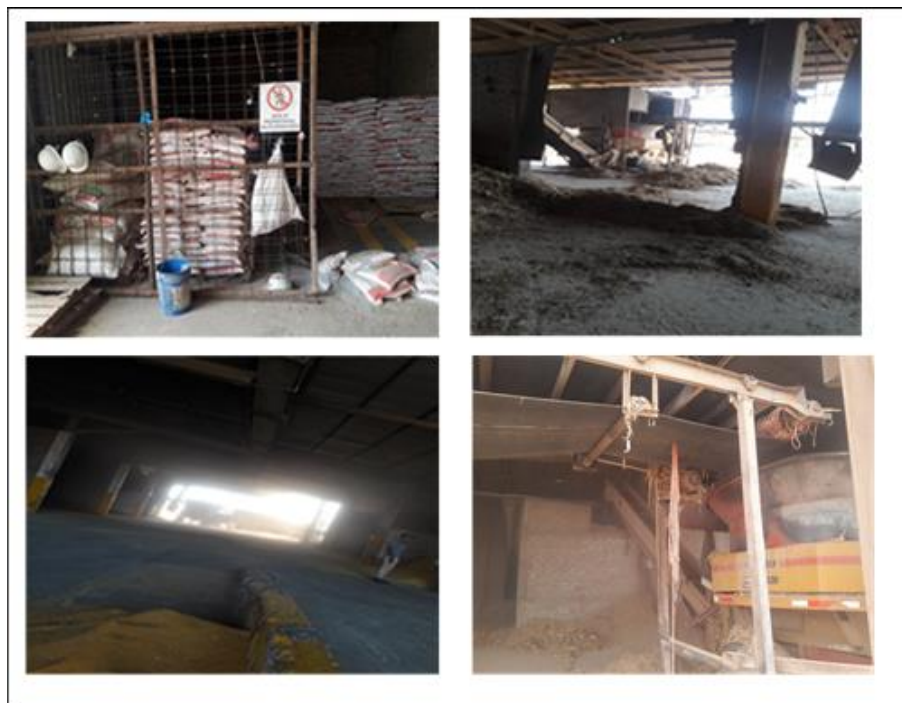
Figure. 1 Current conditions of the food plant
