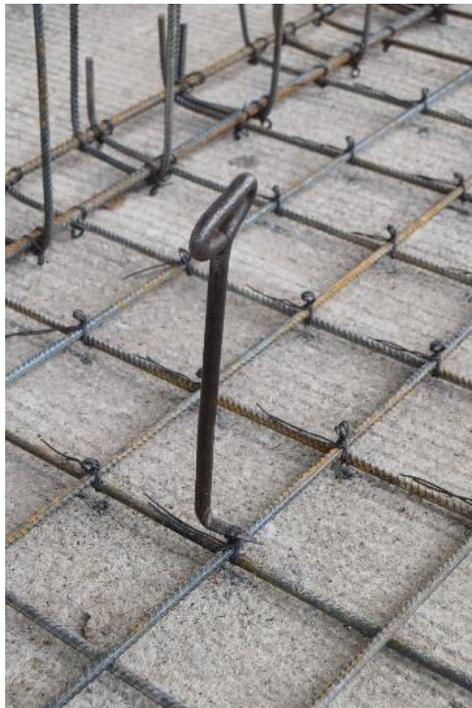
Figure 1 Wire Mooring tool used in the construction site.
