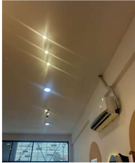
Figure 10. Evidence of ventilation
